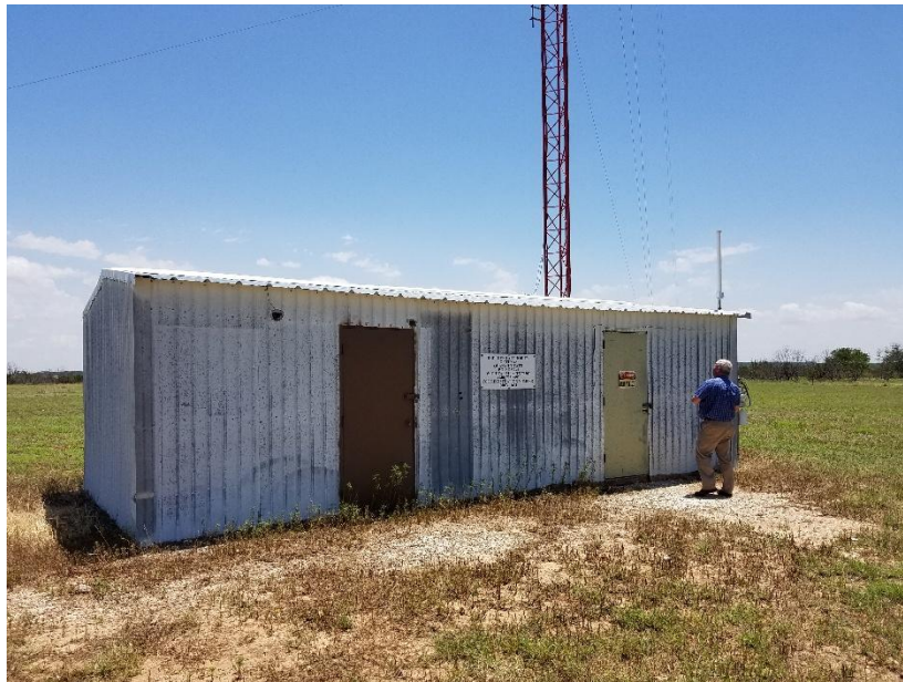
Quanah Tower Communication Building
