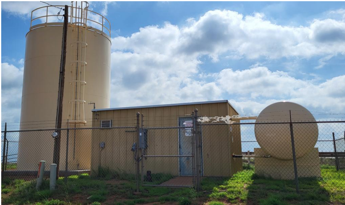
Airport Pump Station – Rehabbed 2023
