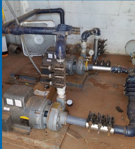
New Pump/Motors Airport Booster
